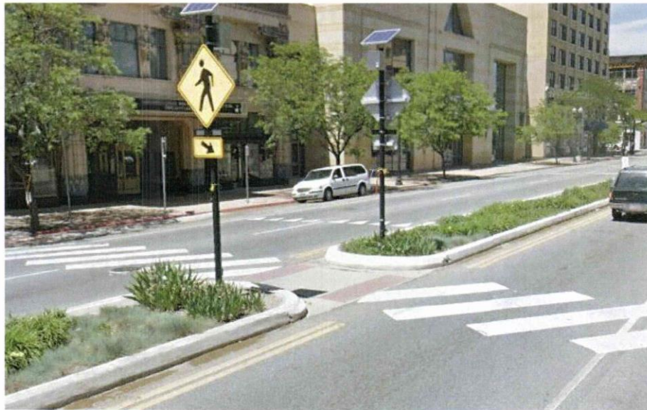
Stamped Concrete Ped Island
