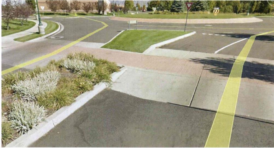
Stamped Concrete Ped Crossing
